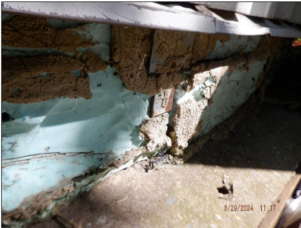
Photo 12 – Exposed Insulation
