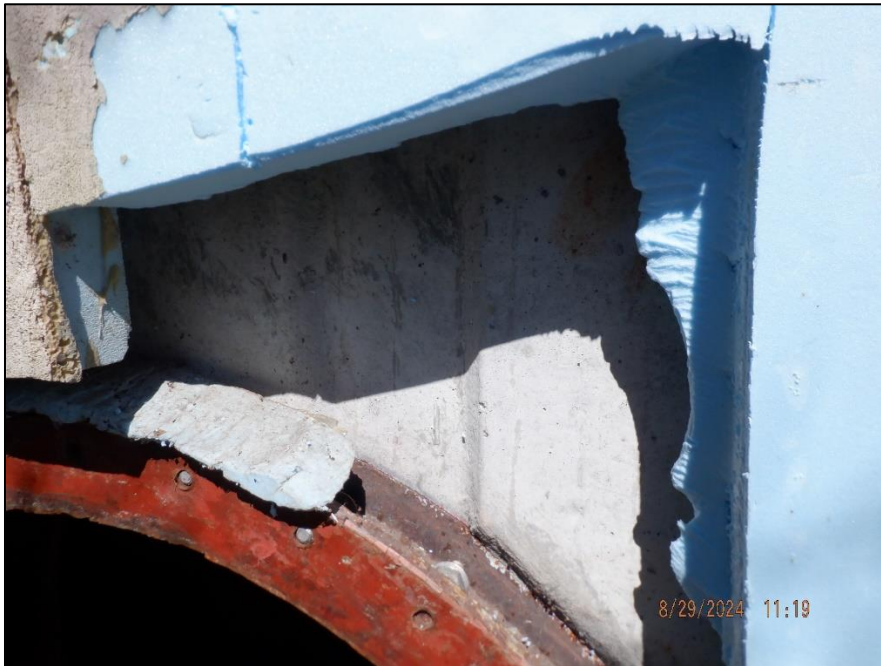
Photo 1 – Wall Assembly at Steel Access Door
