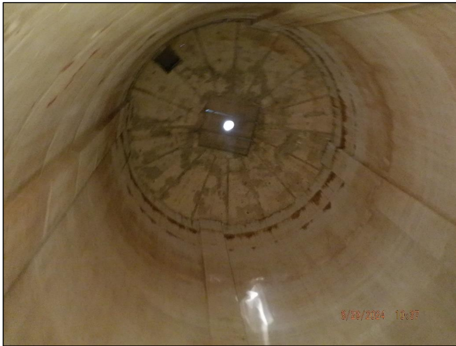
Photo 2 – Interior of Standpipe Tower
