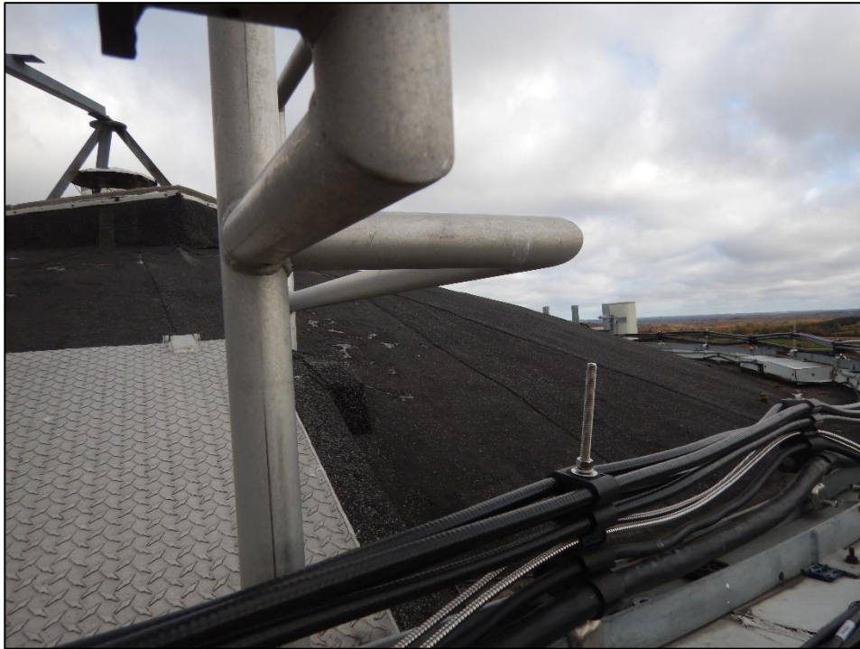
Photo 5 – Roof Structure as seen from Access Ladder
