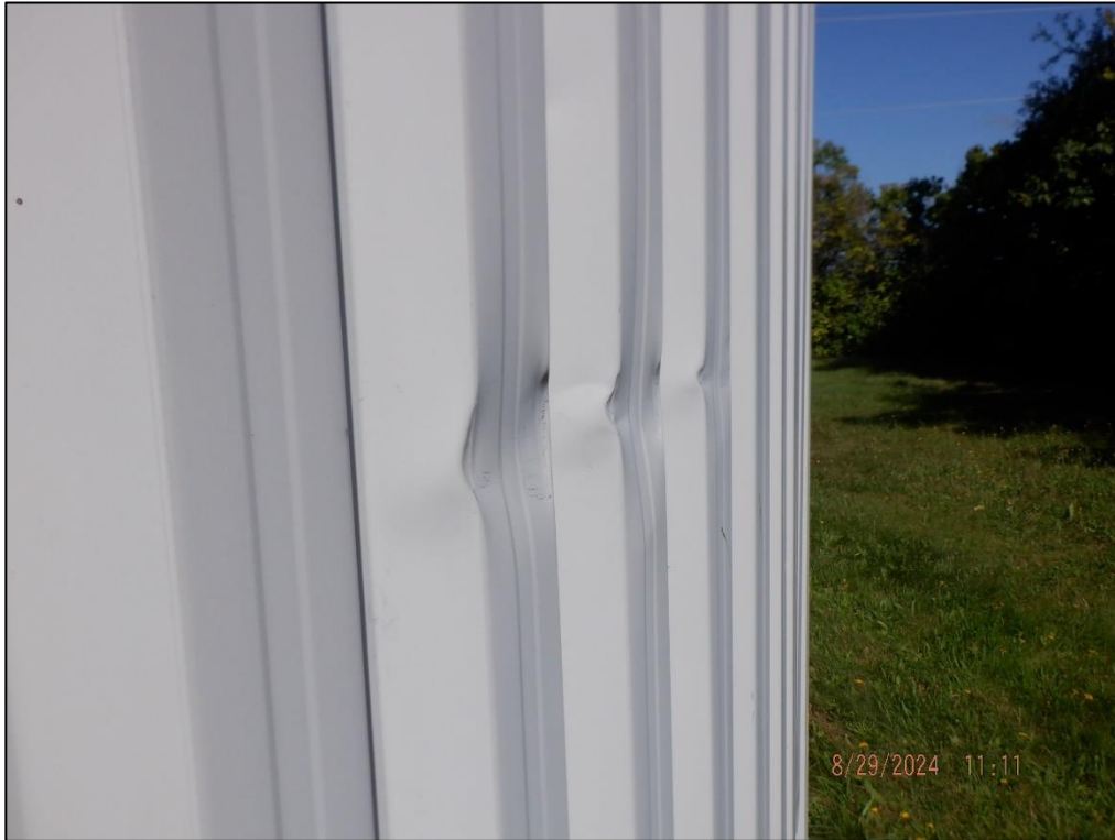
Photo 11 – Deformed Cladding
